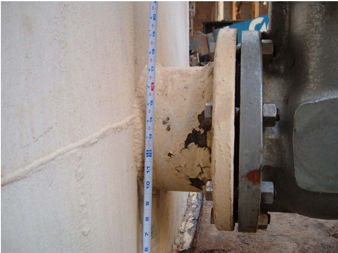
Fig. 2 – Penetration with no reinforcing plate
