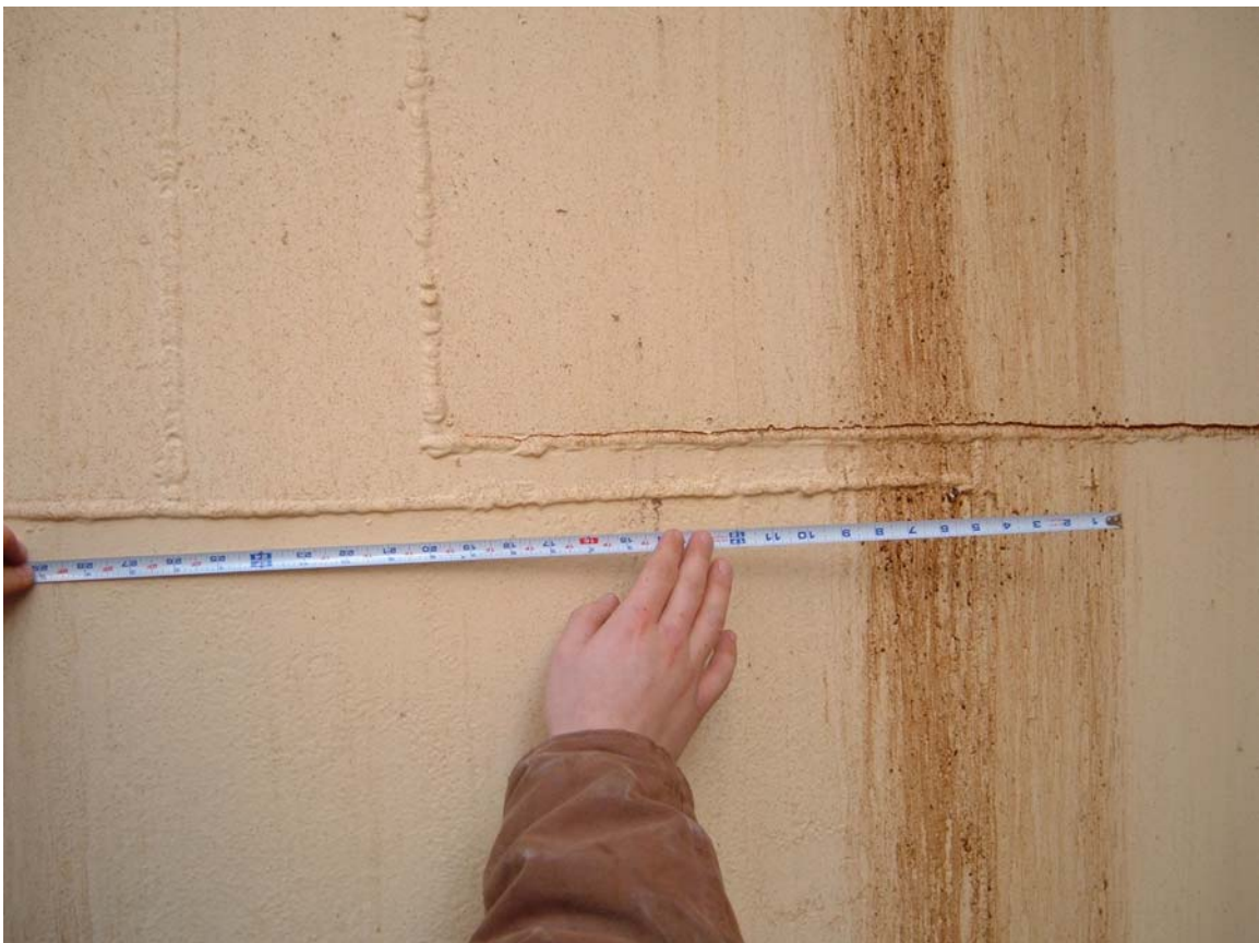
Fig. 6 – Weld spacing does not meet API-650 or good engineering practices
